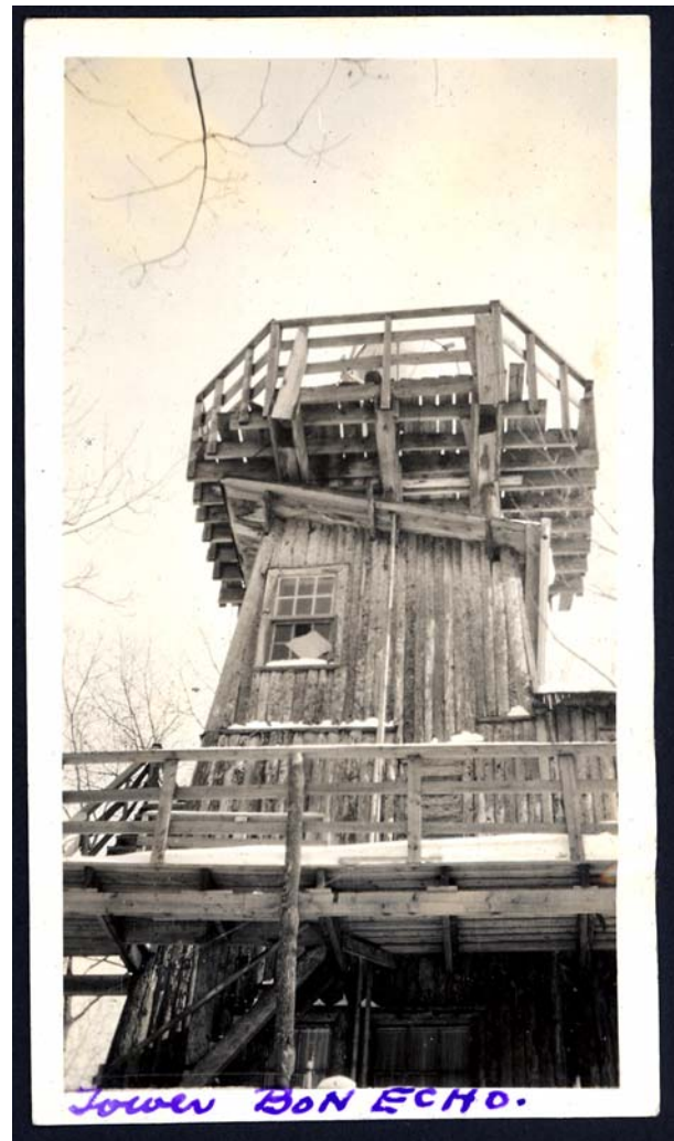
Bon Echo Inn Water Tower
